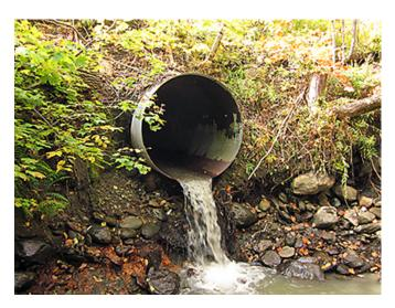
*Fig. 5.4. A road culvert that has been poorly installed, creating a barrier to upstream movement of aquatic life. Credit: Sickter.*
