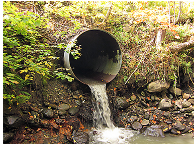
Fig. 5.4. A road culvert that has been poorly installed, creating a barrier to upstream movement of aquatic life. Credit: Sickter.
